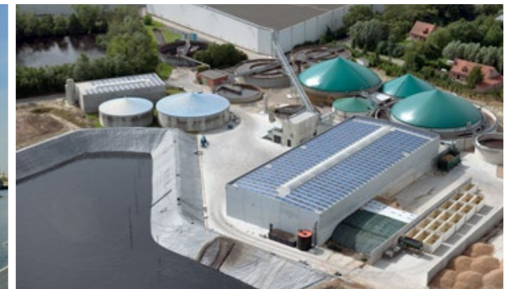
Green electricity and green steam generated at the biomethanisation plant in Ardoorie (BE).
